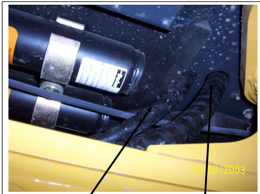
5/16" line going up into the cab.
