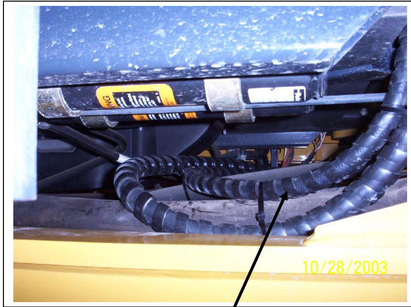
5/16" and 1/2" hoses under the cab looping up towards the existing knockouts in the cab floor on the left side of the cab.
